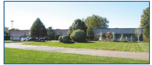
APS's Headquarters in Wallingford, Connecticut
